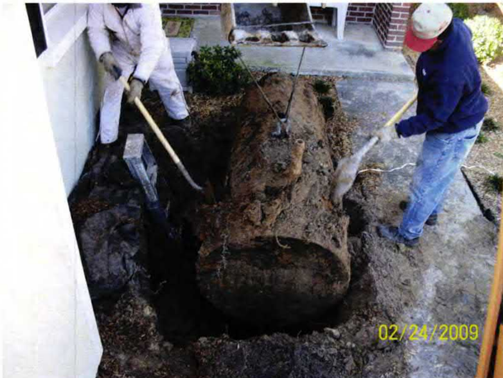
Picture 2: UST 133Banyan during removal.
